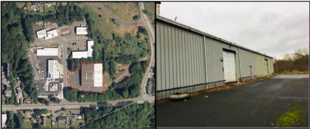
Figure 4: Vacant building at Easter Langlee outlined in red and photograph (Source: BingMaps)
